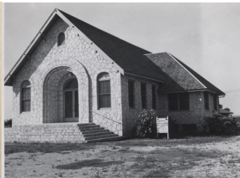
New building after fire
