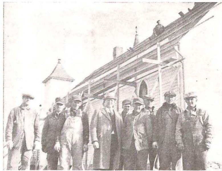
Rev. J. C. Kraenzler (Center) and Members of the Plum Creek Church of South Dakota Who Shingled the Roof of the Church
