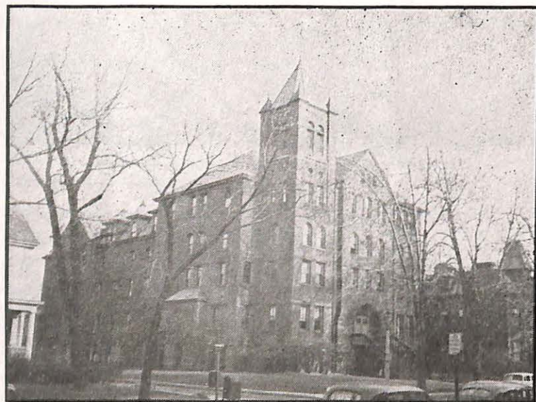
An Unusually Fine View of the Rochester Baptist Seminary Taken by Professor A. A. Schade
