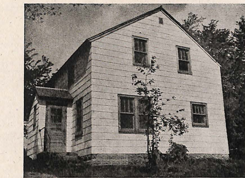
The New Parsonage of the Northside Baptist Church of Hutchinson, Minnesota
