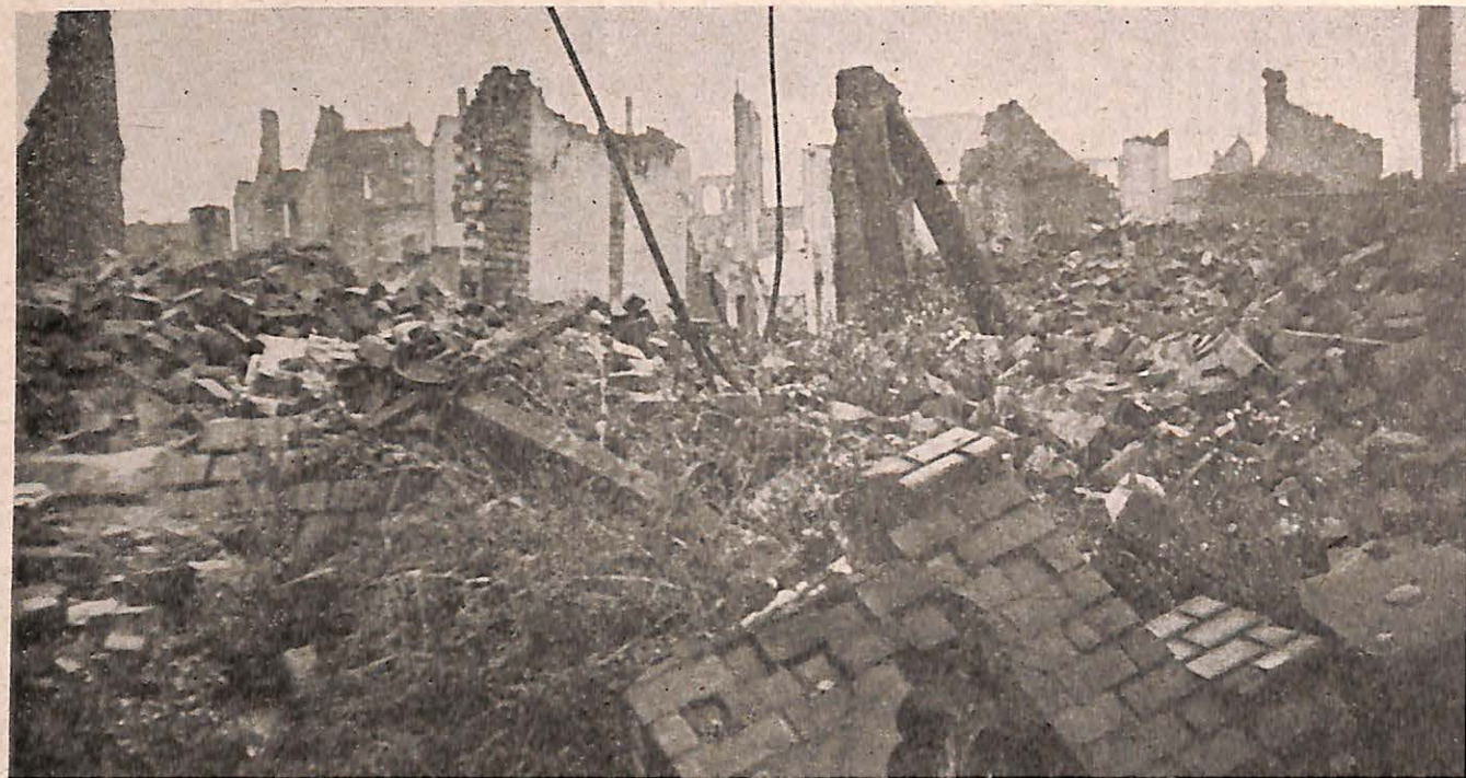
The Ruins of a Baptist Church in One of Germany's Cities, as Photographed by the Rev. William Sturhahn, With the Cross of the Steeple Lying Triumphantly on Top of the Rubble of Bricks
