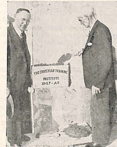
The Laying of the Cornerstone of the New Christian Training Institute Building at Edmonton, Alta., With President E. P. Wahl left and the Construction Superintendent, Mr. Gordon Alexander at Right
