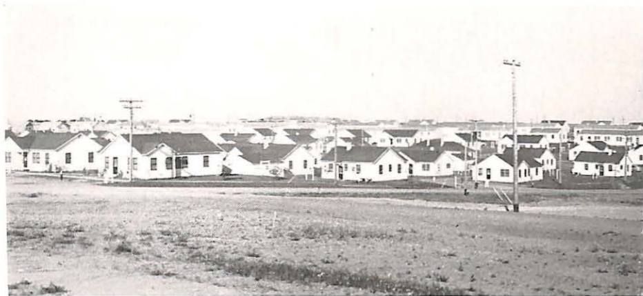
Residential Scene at Garrison Dam in North Dakota Which Shows the Results of Recent "Mushroom Growth"
