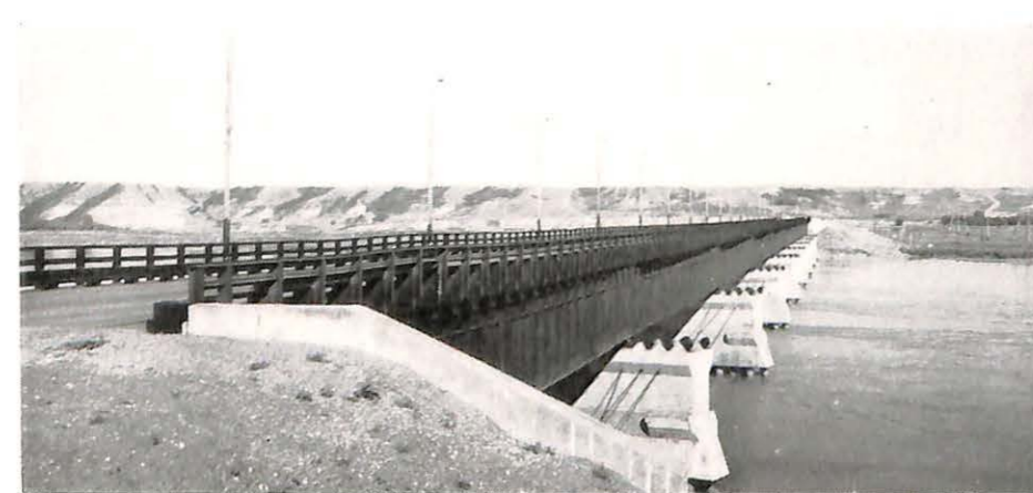
Construction Bridge Over the Missouri River, "The Old Muddy," at Garrison Dam in North Dakota
