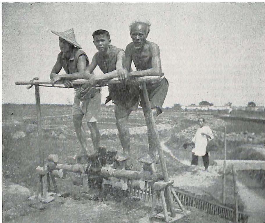
A Chinese "paddy-wheel" or water pump operated by tread-mill to irrigate the rice fields.
