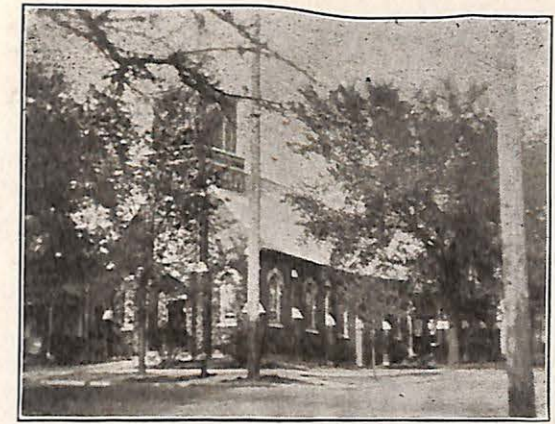
New Building of the Church at Watertown, Wis. Rev. G. Wetter, Pastor
