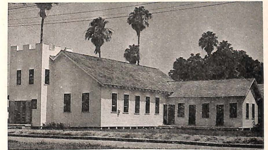
The Enlarged and Renovated Building of the Central Valley Baptist Church, Donna, Texas.
