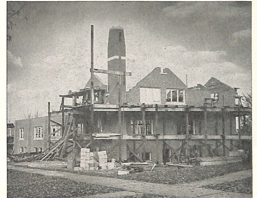
The New Edifice of the Temple Baptist Church, Milwaukee, Wisconsin, Under Construction in November 1948
