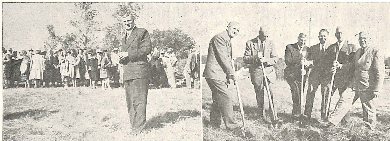
Dr. George A. Lang, President of Our Seminary, as He Calls the Service for the Ground-breaking Ceremonies to Order at Sioux Falls, South Dakota (Left); and the Seminary Building Committee With the Architect (Right) as They Turn Over the Sod During the Impressive Exercises
