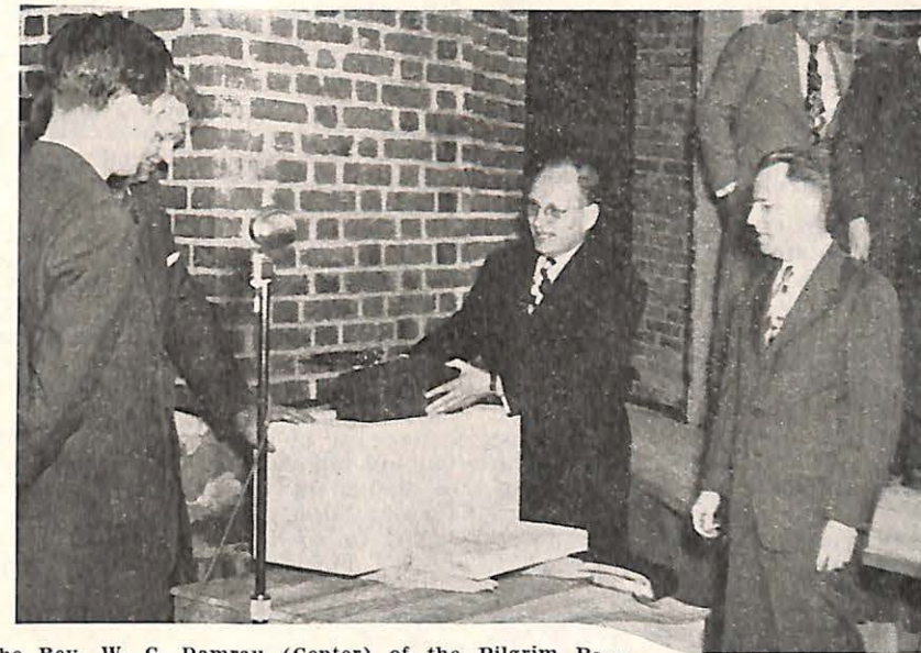
The Rev. W. C. Damrau (Center) of the Pilgrim Baptist Church, Philadelphia, Pa., Placing Objects Into the Cornerstone of the New Edifice Watched by Mr. Otto Draeger (Right) and Rev. John F. Crouthamel and Rev. Frank H. Woyke (Left)
