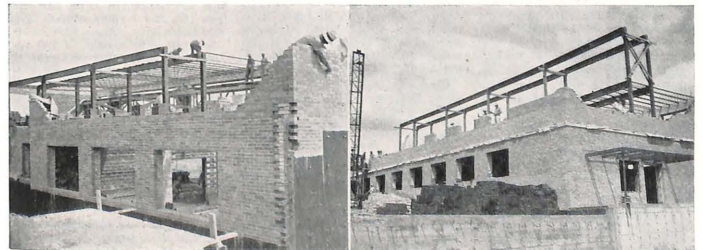
Work is progressing rapidly on the new buildings of the North American Baptist Seminary, Sioux Falls, South Dakota, as seen in the dormitory wing at the right and in the administrative building on the left
