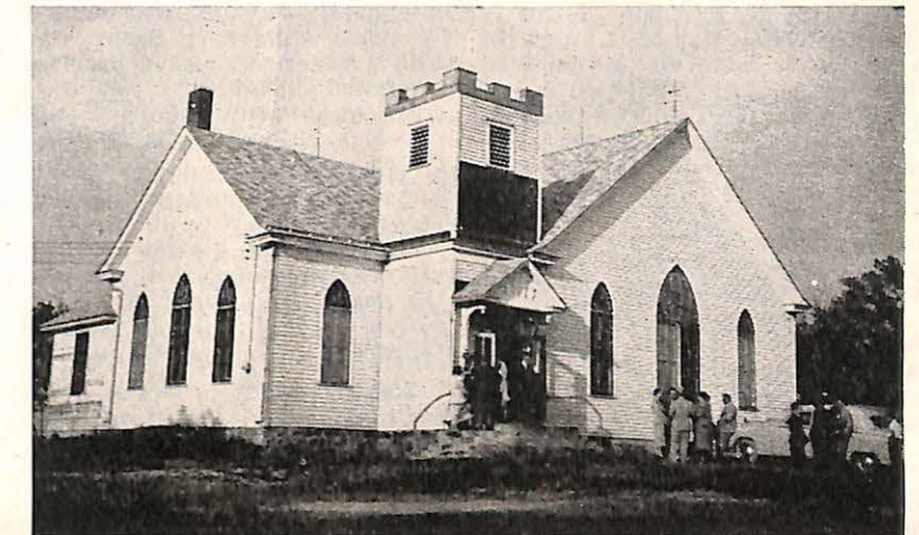
The edifice of the Dickinson County Baptist Church near Elmo, Kansas, with the reconstructed steeple (not painted as yet). The Rev. Herbert Schauer is the pastor.
