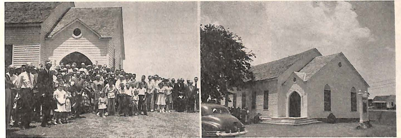
On Sunday, May 20, the remodeled edifice of the Greenville Baptist Church near Burton, Texas (right), was rededicated and many members and friends from sister churches in Texas gathered to celebrate the 90th anniversary of the Greenville Church, the oldest church in the Southern Conference.
