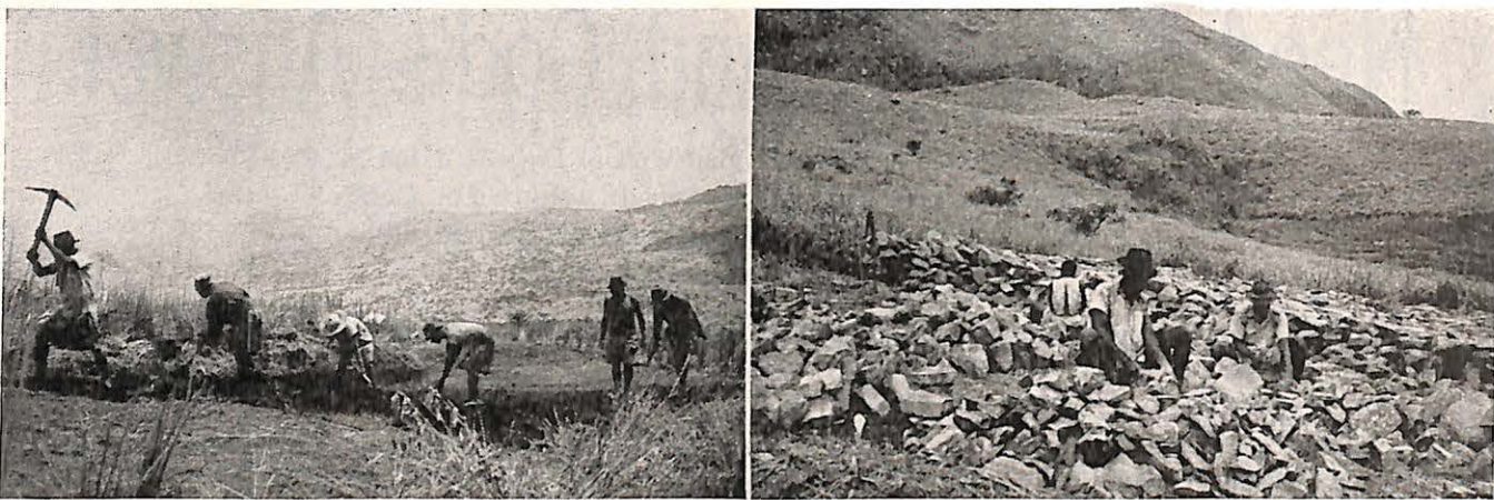
Digging for the foundations and preparing the stones and rocks for the new buildings of the Bamenda New Hope Settlement, our new leper camp in the Cameroons, Africa.
