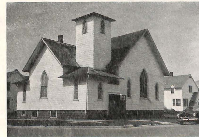
The newly purchased and rededicated edifice of the First Baptist Church, Sumner, Iowa, which was formerly a United Brethren Church.
