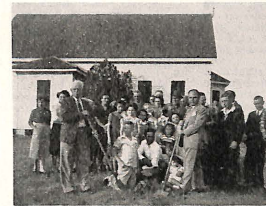
Ground breaking exercises for the new edifice of the Mowata Baptist Church, Branch, Louisiana, with the Rev. Alex Sootzmann, pastor, at right with the shovel surrounded by members and friends of the church.
