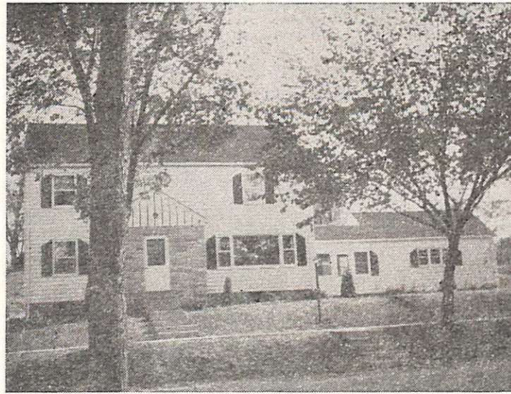
The new parsonage of the Baptist Church, Aplington, Iowa, in which the Rev. and Mrs. Frank Veninga and their family have been the first occupants
