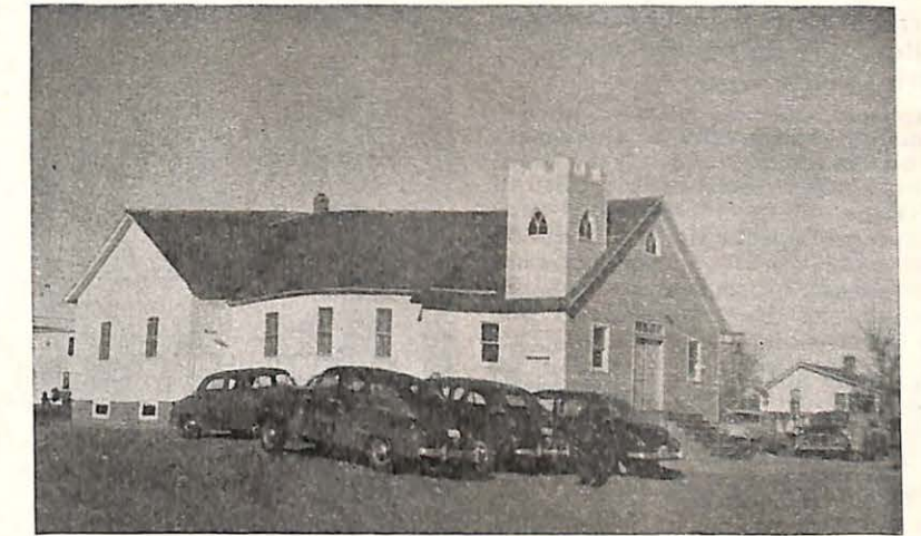
The remodeled edifice of the Baptist Church, New Leipzig, North Dakota, which was recently rededicated.
