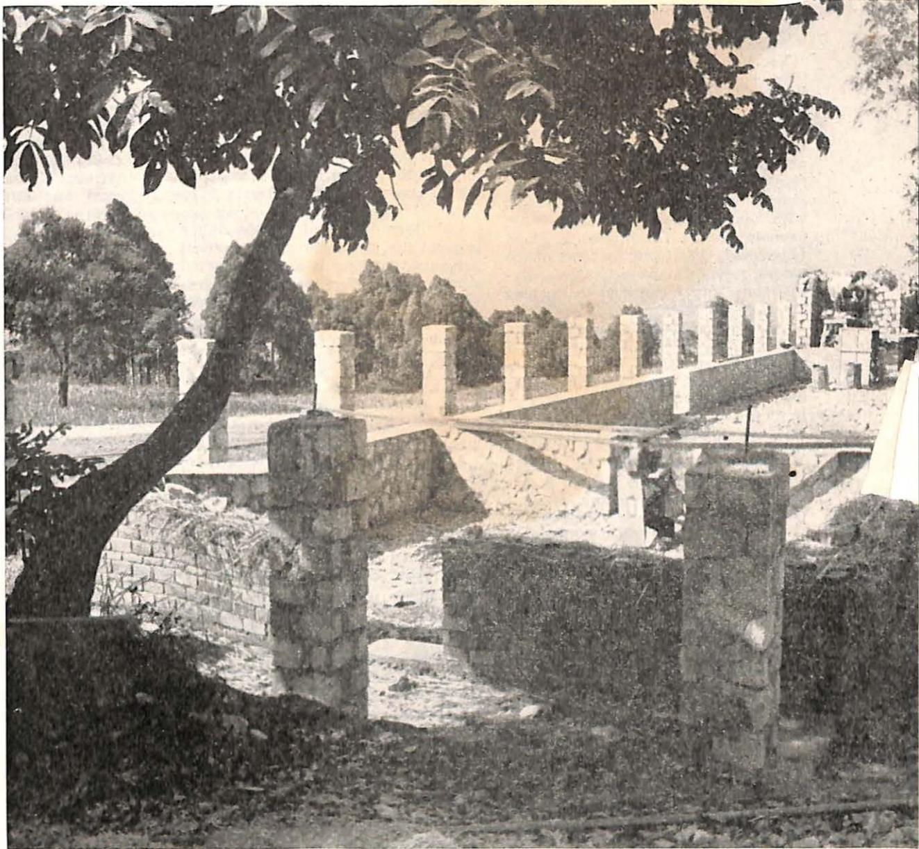
Thirty Bed Ward at the Banzo Hospital Under Construction
