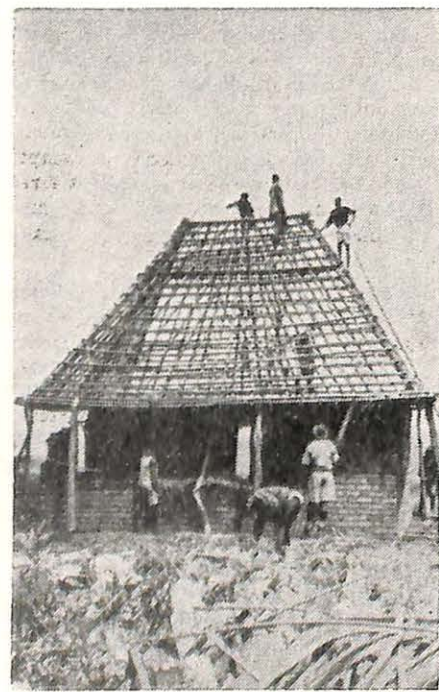
Leprosy patients working on the roof of the New Patients' Quarters at the Bamenda New Hope Settlement
