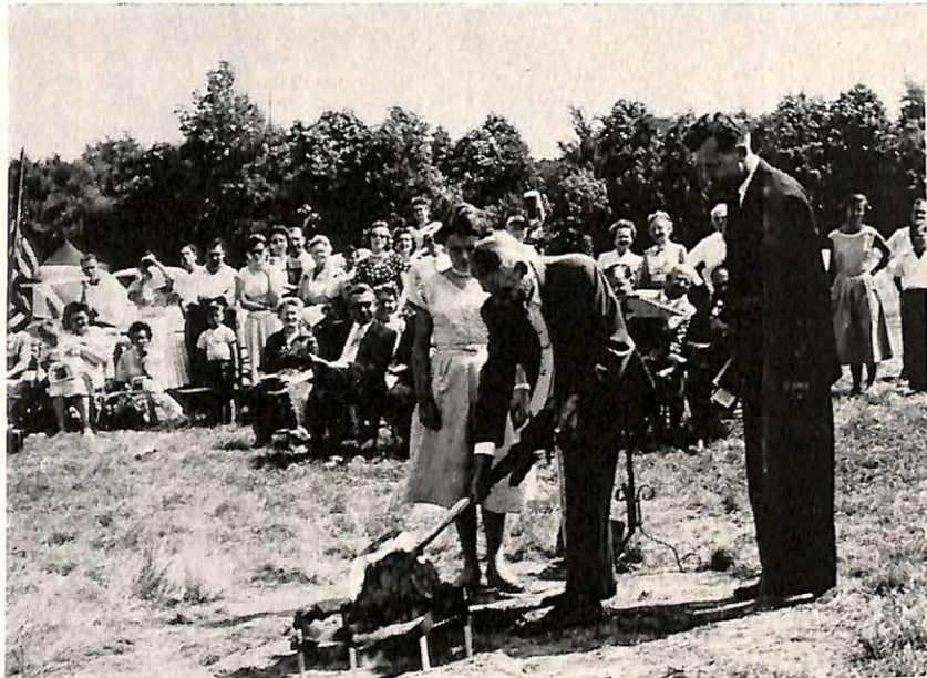
Ground breaking exercises for the Parma Heights Baptist Church, Parma Heights, Ohio with the Rev. Edwin Miller, pastor, standing at the right; Mr. Berthold Hemme, honorary deacon, turning over the first shovel full of ground; and Miss Eleanor Ludwig who presented the shovel to each participant in the ground breaking ceremony
