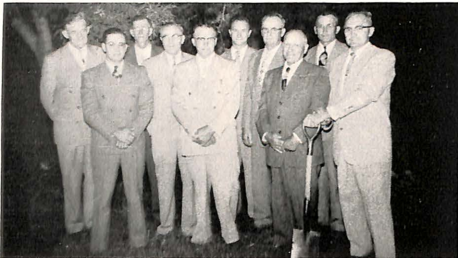
Rev. A. J. Fischer (right), pastor of the Baptist Church, Linton, N. Dak., and deacons of the church and the building committee at the ground breaking exercises for the new parsonage.
