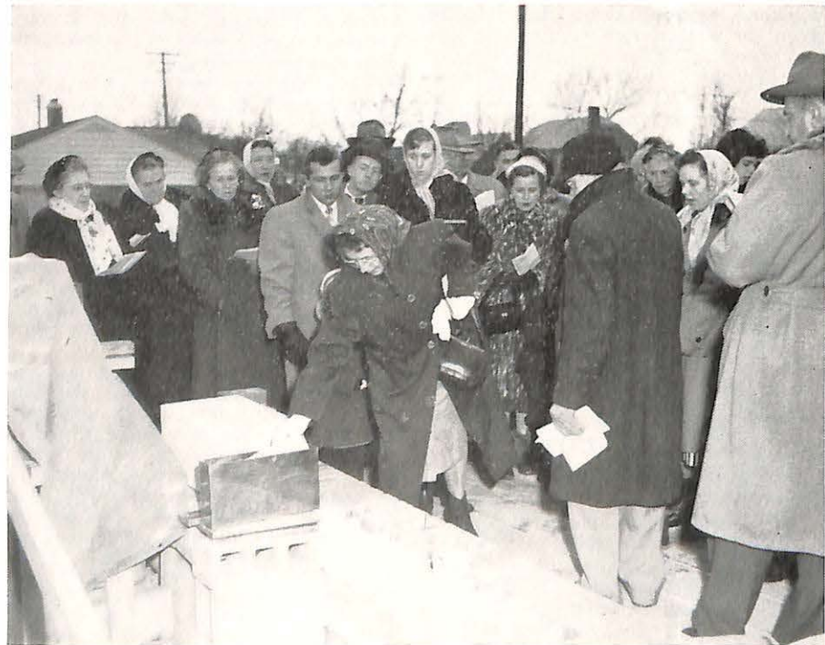
The cornerstone of the new First Baptist Church, North 11th Street and Waldo Blvd., Manitowoc, Wis., was set in place during special ceremonies, Sunday morning, December 4th. In the picture, Mrs. Henry Specht, is placing denominational literature and church newspaper clippings in the copper box which was sealed into the cornerstone. George Anhold (right), a deacon, placed a copy of the church covenant and constitution in the box. Rev. Harvey Rakow (far right), conducted the service. Participating were George Specht, deacon; Erwin Anhold, building committee; and Fred Rauber, architect.
