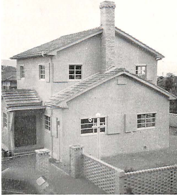
The new Baptist Mission House in the Kinkakuji area of Kyoto, Japan.
