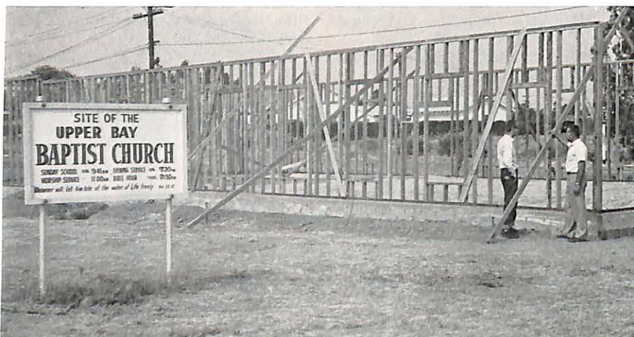
The Upper Bay Baptist Church, Santa Ana Heights, Calif., under construction. Rev. Fred David is pastor of this Church Extension project.
