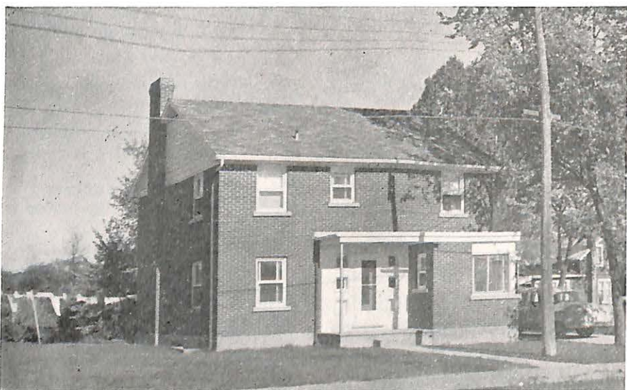
The new 8-room house and parsonage of the First Baptist Church, Arnprior, Ontario, Canada, which was recently dedicated.
