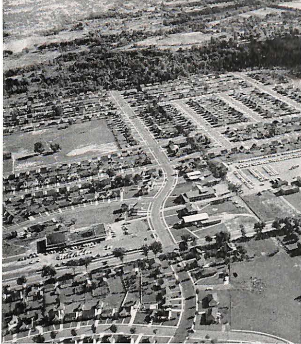
An airplane view of beautiful Colonial Village, Lansing, Mich., showing the Colonial Village Baptist Church to the right of Boston Boulevard (almost at center of photograph alongside the board street).
