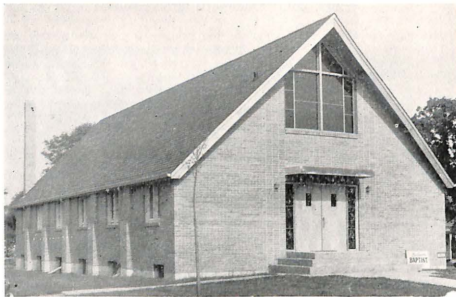
The new edifice of the Bethany Baptist Church, Hutchinson, Minn., which was dedicated on Sunday, June 16, 1957.
