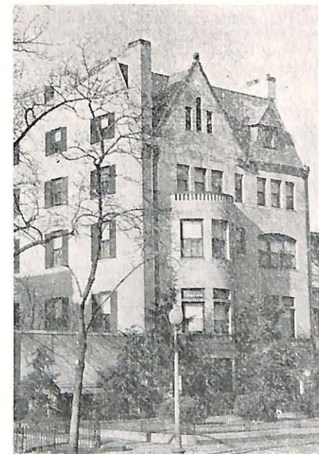
Offices for the Baptist Joint Committee on Public Affairs are in this Washington, D. C., building. Here members of this North American Baptist General Conference agency work to preserve religious liberty and separation of church and state in our country.
