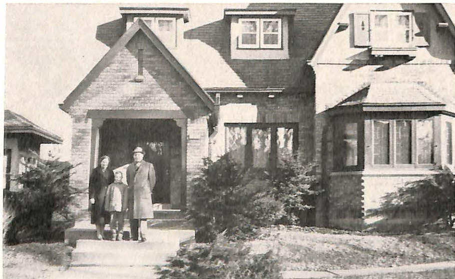
ZION CHURCH PARSONAGE, MILWAUKEE, WIS.
