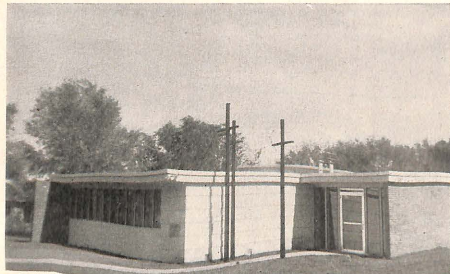
The newly dedicated edifice of the Bethel Baptist Church, Cherokee, Oklahoma. Rev. Kenneth E. Unruh is the pastor of the church.
