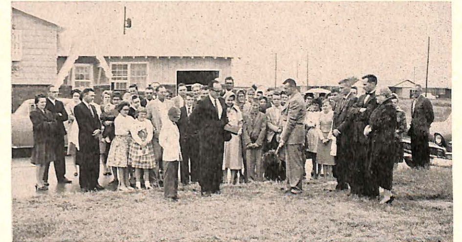
At the ground breaking exercises held by the Memory Lane Church, Wichita, Kansas, Mr. Reid Storey (with spade), Trustee-Building Committee chairman, began the ceremony. Behind him are Fred Savage, Terry Storey and Mrs. Rose Berger, members of the Trustee-Building Committee.
