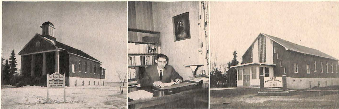
The First Baptist Church of Leduc, Alberta, built in 1928 (left) before present renovation, and the new church building in 1961 (right) at the Dedication Service. Rev. Paul Siewert (center) is the pastor.
