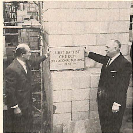
Cornerstone laying exercises for the Educational Building, First Baptist Church, Lodi, Calif.
