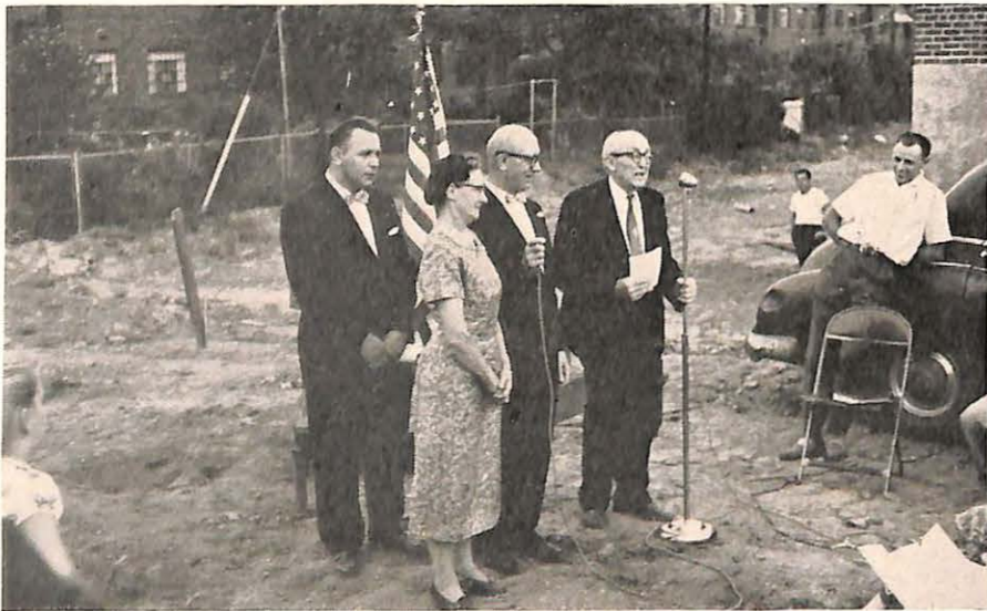
Groundbreaking service held by the Immanuel Church of New York, N. Y., at its new church site in Woodside, Long Island.
