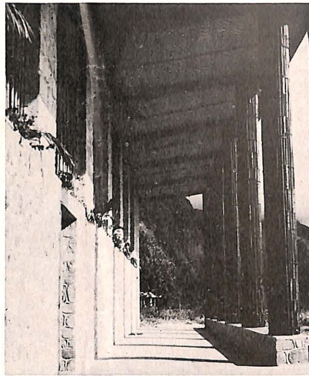
The veranda and entrance (left) to the newly dedicated New Hope Settlement Church at Mbingo in West Cameroon, showing the bamboo covered pillars, the lattice-work windows and woven mats on the ceiling planned by Missionary Gilbert Schneider.
