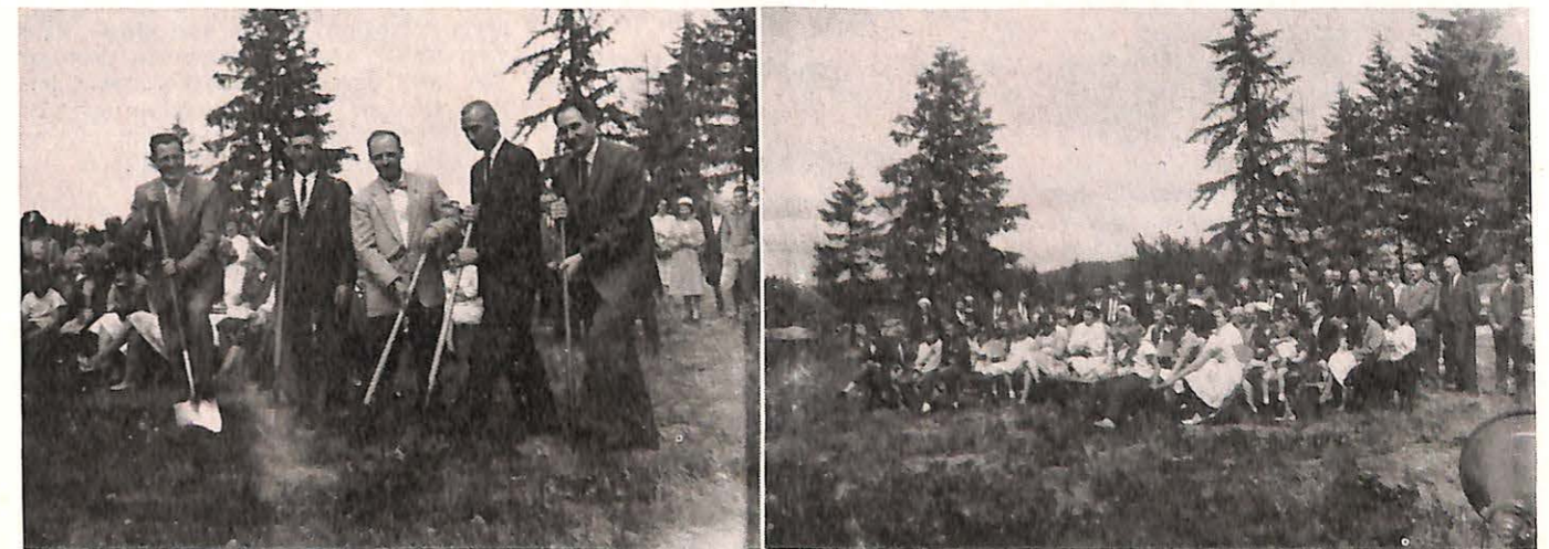
Ground breaking service held by the Sierra Heights Baptist Church, Renton, Wash., on Sunday, June 17th, with church leaders, including the pastor, Rev. Ervin Gerlitz (left), using the shovels and with the large crowd of members and friends in this beautiful out-of-door setting.
