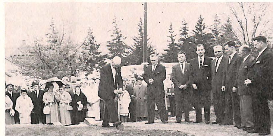
Ground breaking exercises for the new $250,000 building project of the Baptist Haven of Rest for the Aged, Medicine Hat, Alberta. Construction on the new building is now under way.
