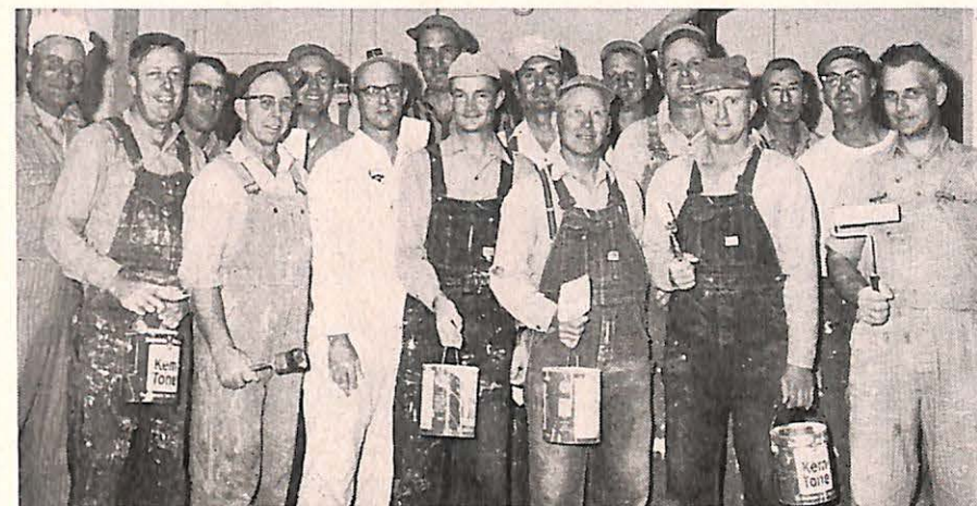
Men of the First Baptist Church, Lorraine, Kansas who "contributed" a day to paint and do repair work on the building of the Calvary Baptist Church, Hoisington, Kansas.
