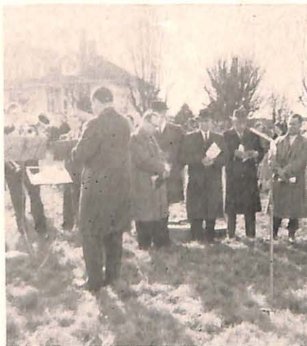
Ground breaking exercises by the Rose of Sharon Baptist Church, Richmond, British Columbia.
