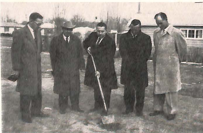
Ground breaking service for new South Canyon Baptist Church, Rapid City, S. Dak. Left to right: Mr. Alvin Auch, Mr. Everett Crooks, Rev. W. D. Dachtler, pastor; Mr. Miles Taggart, contractor; and Mr. John Kwyzla.
