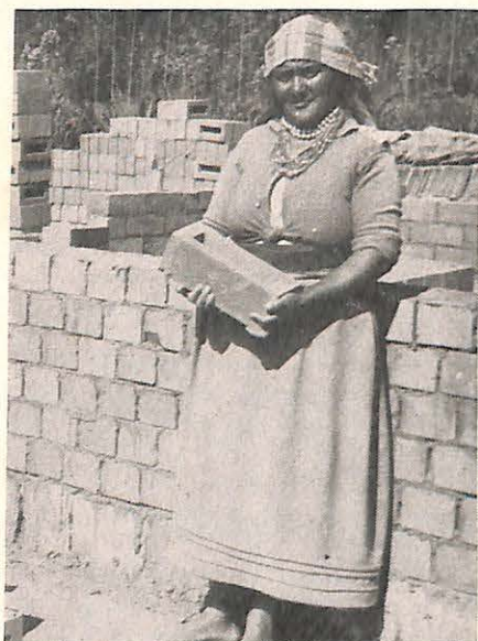
An Indian woman with her family building a mud brick house at Calderon, near Quito, Ecuador.
