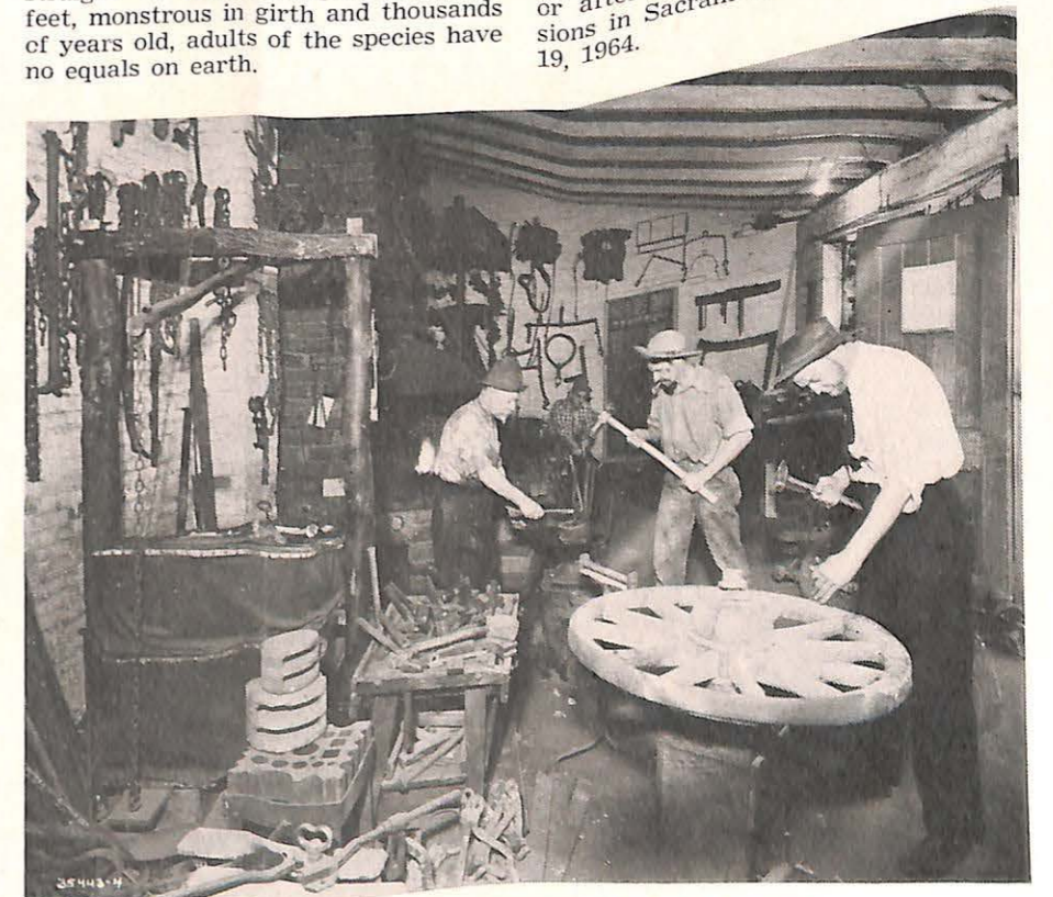
BLACKSMITH SHOP AT SUTTER'S FORT, SACRAMENTO Here in this reconstructed Blacksmith Shop in Sutter's Fort, one can see many old tools of the California pioneers, a forge with its great hand-made bellows, and the innumerable sooty objects to be found in these old shops.
