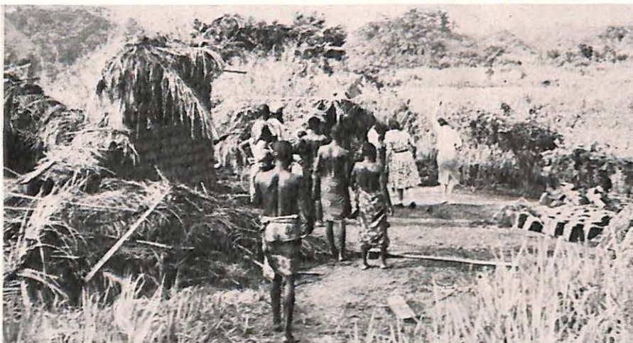
A new Baptist Church building is begun at Obang in the Wum division as "everybody came to help and to build together for Christ." (Photo by Laura E. Reddig).
