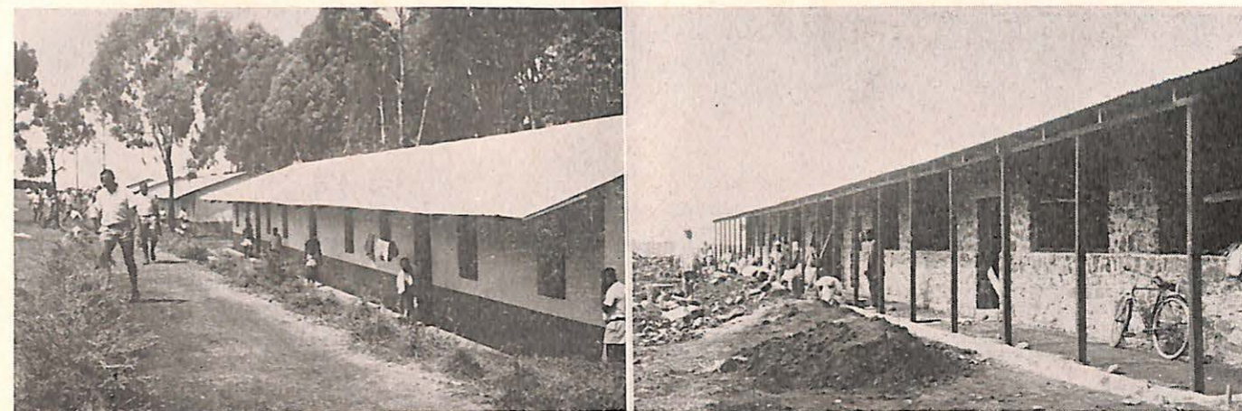
Several dormitories and one dining hall of the Ndu Baptist College are shown in this picture (left). They are built entirely of mud block. At the right, the new four classroom block is under construction.
