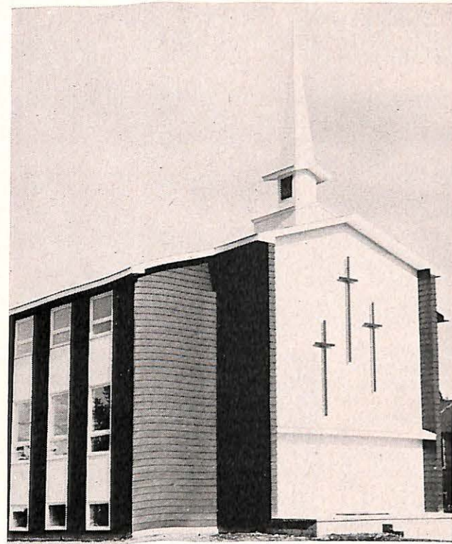
Grandview Baptist Church of Anchorage, Alaska built with volunteer help and with a Baptist builder from Texas serving as foreman on the job.
