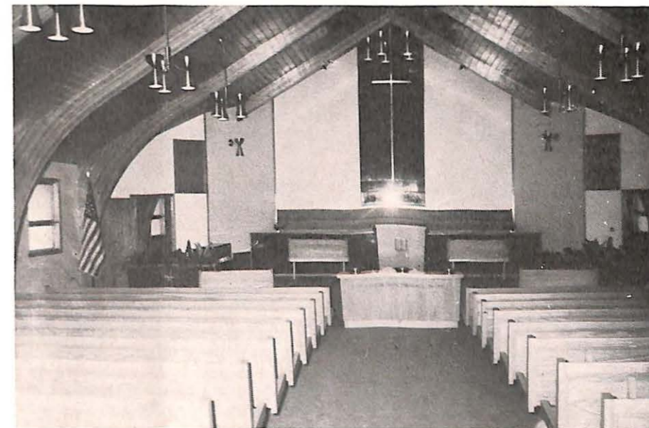
The new sanctuary of the Venturia Baptist Church, Venturia, North Dakota built largely with volunteer labor under the supervision of Rev. M. W. Falkenberg, pastor, as architect and contractor.
