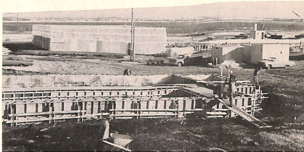
Base for the boys dormitory in the foreground and the administration unit to the center left.
