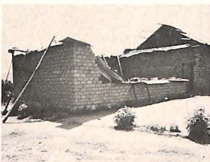
Warwar photo—H. Johns New school under construction.
