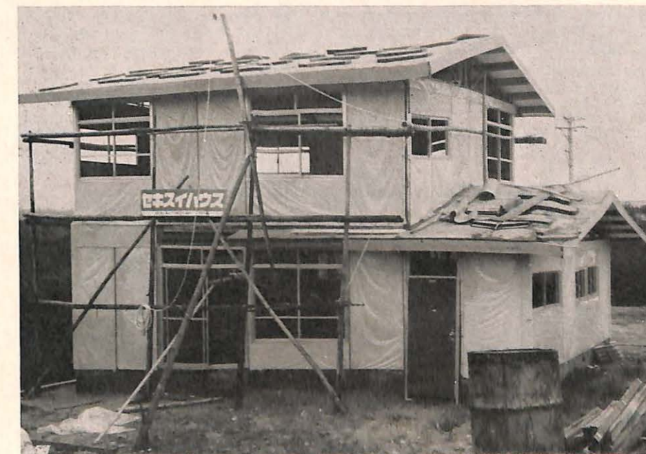
Construction on the new house in Nagoya, Japan. Rev. and Mrs. Edwin C. Kern moved to Nagoya in May to begin evangelistic work.
