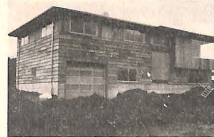
Parsonage in construction on church property.
