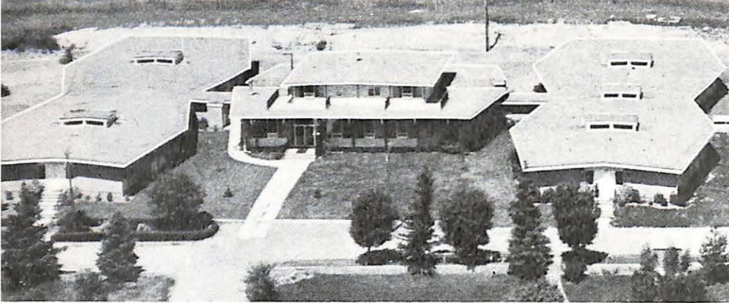
In 1962 the present facilities of the Baptist Haven of Rest, Medicine Hat, Alta., were built.
